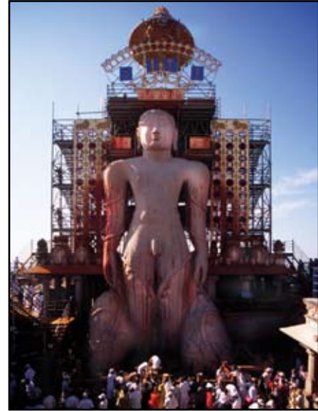
Scaffolding has been constructed around the statue of Bāhubali in preparation of the great ritual.
